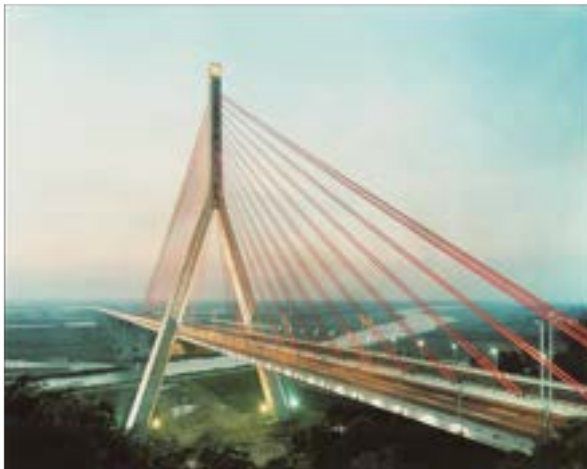
Chun Yu Structural Bolts are deployed on the "Kaoping Cable-Stayed bridge".
